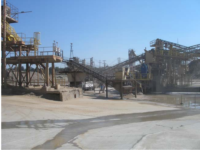
Figure 2-21. Process Equipment Upwind Monitors Looking Toward Conveyor Transfer Point, Vibrating Screen and Crusher, Carroll Canyon
