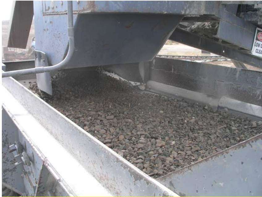
Figure 2-6. View of Vibrating Sizing Screen Material Inlet, Barstow
