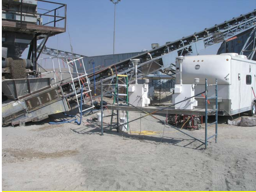
Figure 2-10. View of Transfer Point and Upwind PM 4 Monitors, Barstow
