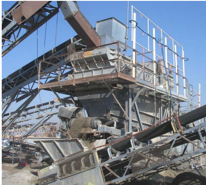
Figure 2-5. Side View of Vibrating Sizing Screen Array, Barstow
