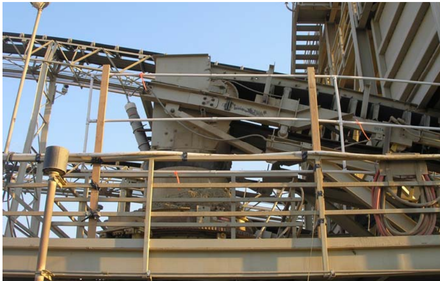
Figure 2-26. Side View of Upper Crusher Array, Vernalis
