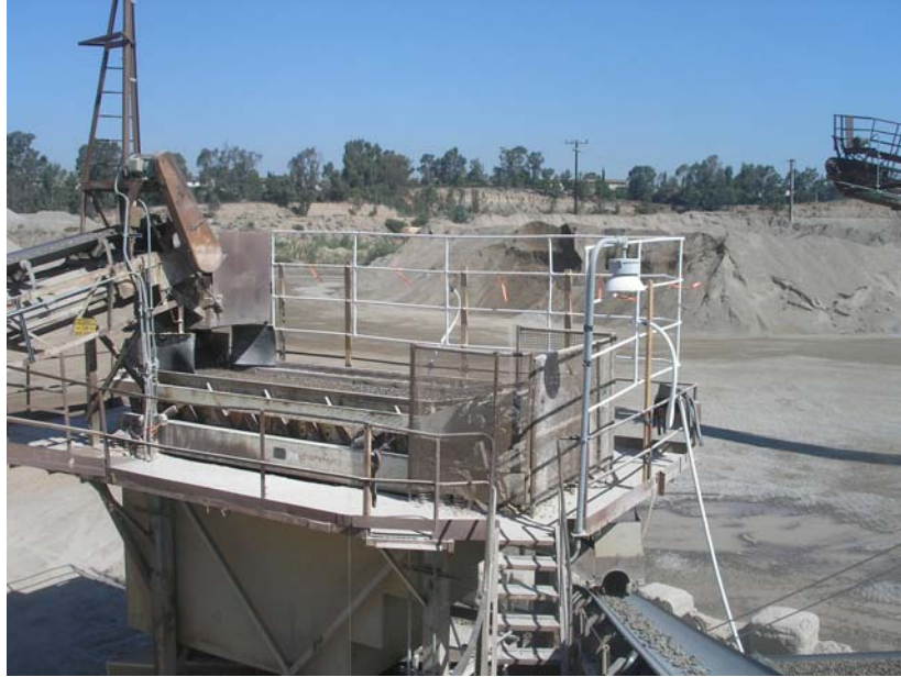
Figure 2-13. Side View of Vibrating Sizing Screen Array, Carroll Canyon
