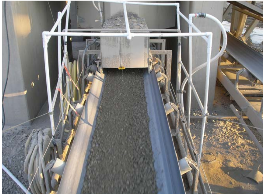
Figure 2-27. Side View of Crusher Material Outlet, Vernalis
