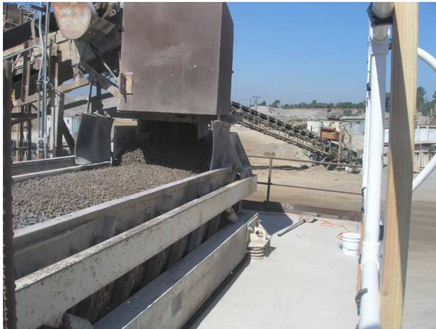
Figure 2-14. View of Vibrating Sizing Screen Material Inlet, Carroll Canyon
