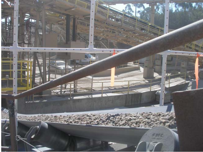
Figure 2-19. Close Up View of the Conveyor Transfer Point Upper Array, Carroll Canyon
